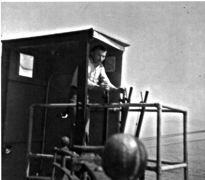
The author, in 1956, on the controls of boom landing men and supplies on the lighthouse. Author's collection.
